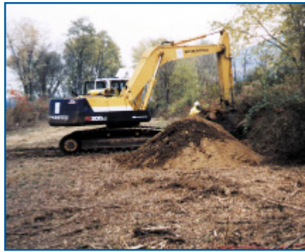
KEY has completed long-term monitoring in support of soil remediation projects.
