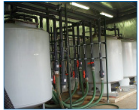
KEY has designed carbon treatment systems that include access points for collection of discrete air samples.
