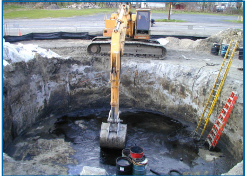
Manufactured Gas Holder Remediation
