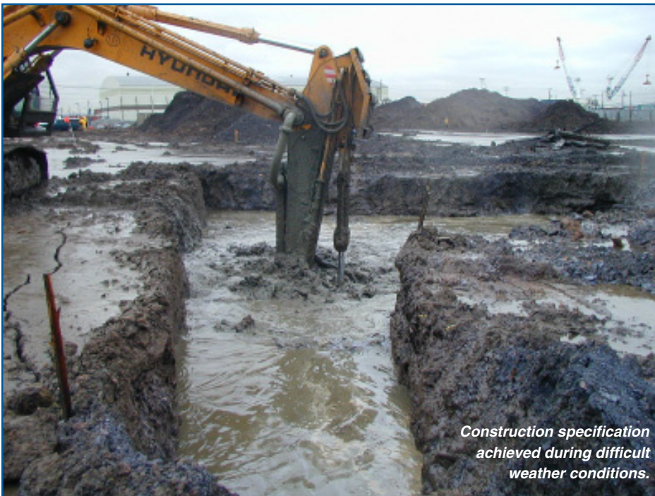
Mixing head for deep stabilization.
