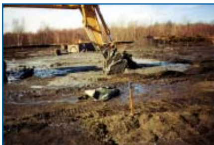
Cement-soil mixing operations using the Lang Tool, LTC-290 mixer/blender.
